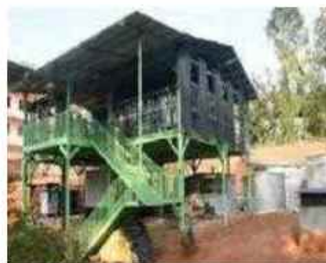
1 MLD STP at Kozhikode medical College
